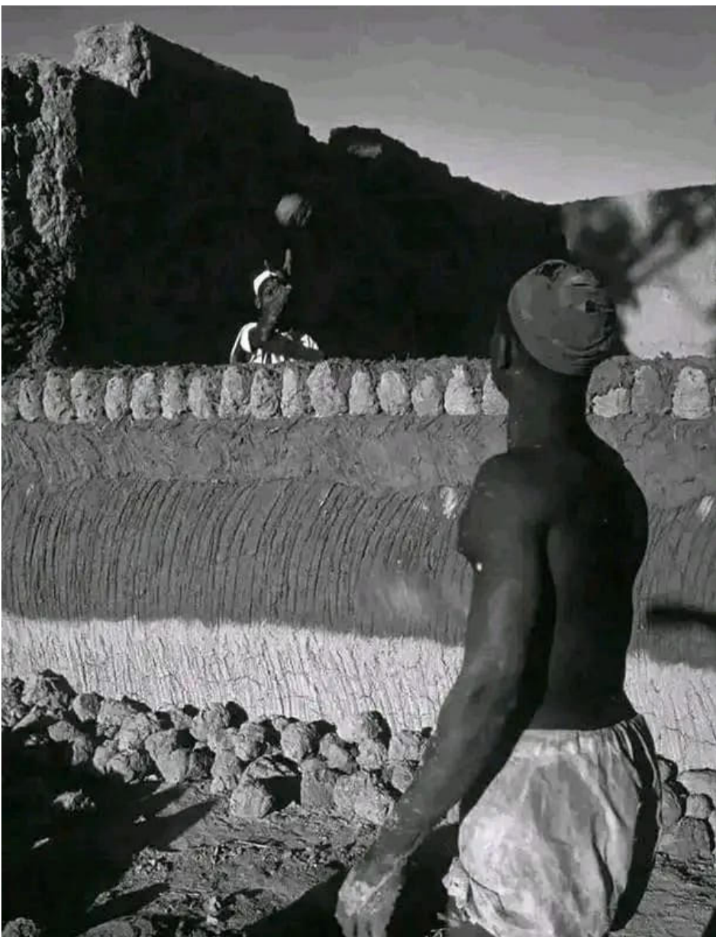
A photograph of Hausa builders constructing a mud (tubali) fence in a community within Katsina State in 1957.
